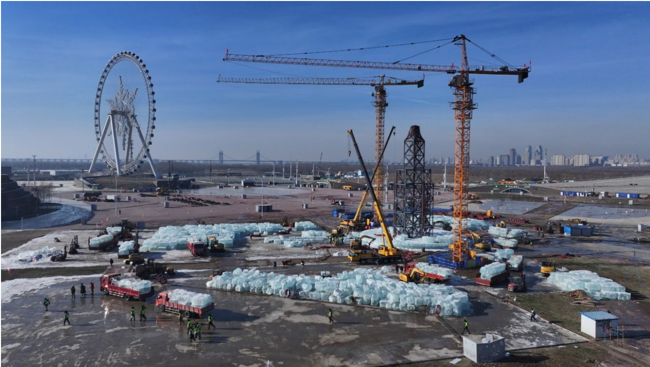
Figure A.18 Construction and Building-1
