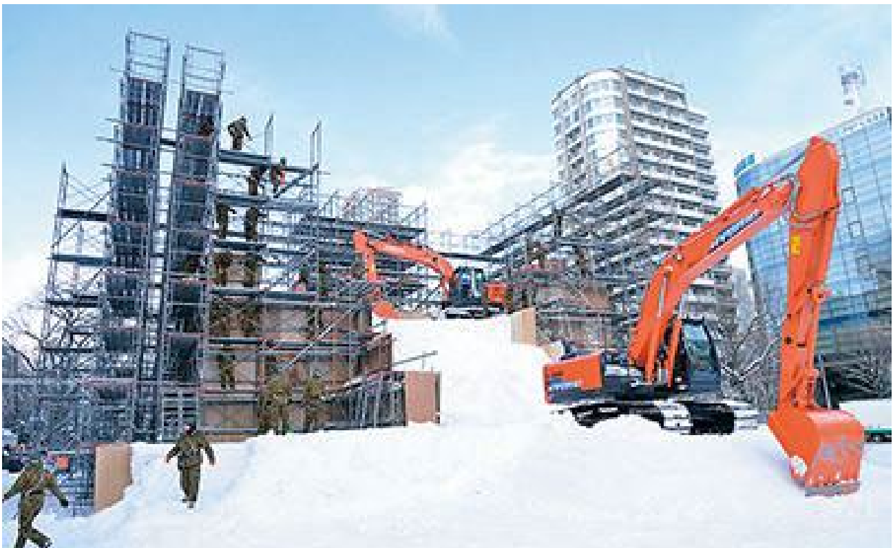
Figure A.10 Construction and Building-1
